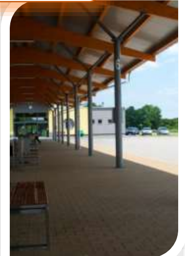
Somewhere to sit and shelter whilst waiting for a bus or train.
